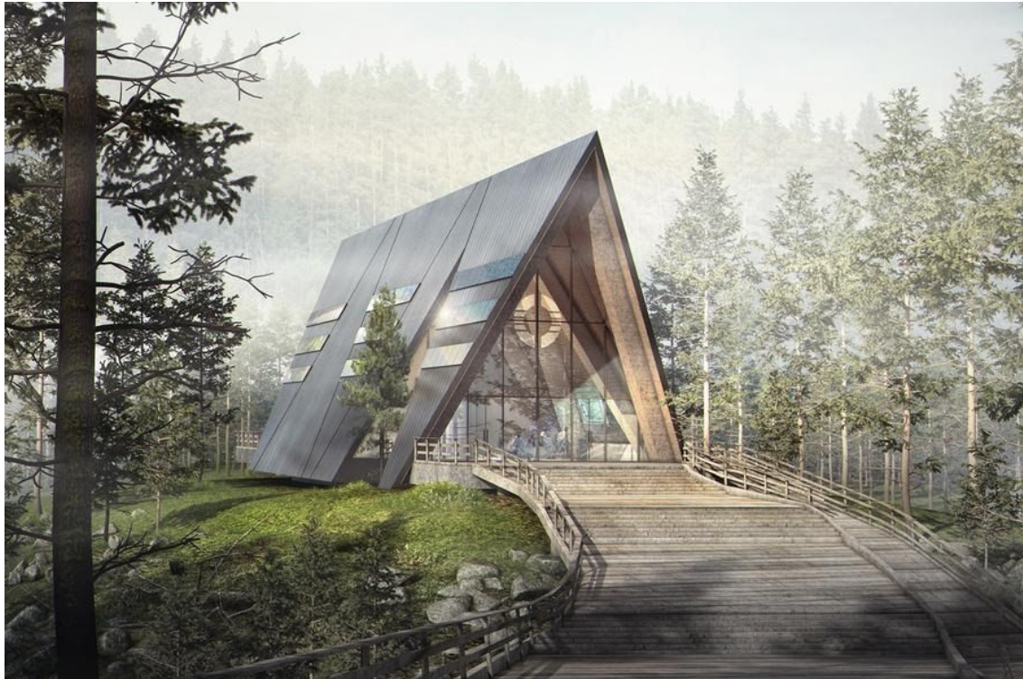
Figure 2.3. An artist rendering of the Aurora, Oklo's 1.5 MW MNR design. With a small footprint and a reactor installed below grade, this system bears little resemblance to a conventional nuclear plant. (Image courtesy of Oklo).
